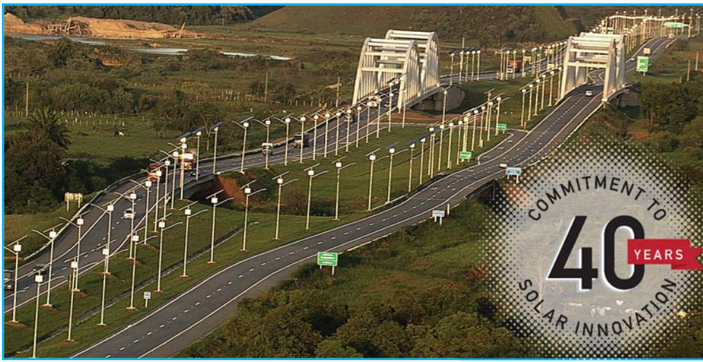
THAT'S INNOVATIVE: About half of Brazil's new 145-kilometer Arco Metropolitano highway is illuminated at night by solar streetlights, powered by Kyocera PV modules — 3.2 megawatts in total.
